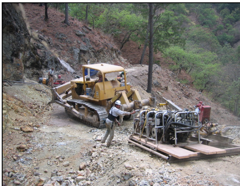
Drilling at Reventon Breccia
