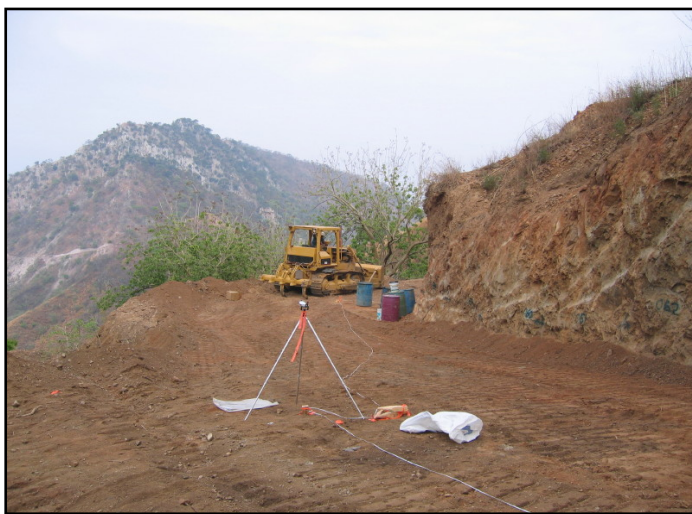
Trenching at the San Rafael Zone
