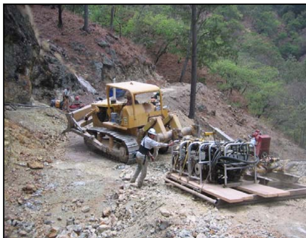
Drilling at Reventon Breccia
